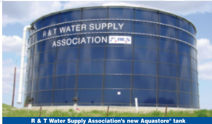
R & T Water Supply Association's new Aquastore® tank
