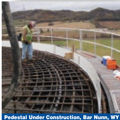
Pedestal Under Construction, Bar Nunn, WY
